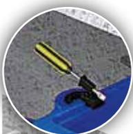
The electrical cables are passed through special patented cable glands that ensure a perfectly watertight seal. Before fitting the cable, perforate the cable glands to be used with a sharp tool, but leave the others intact to keep liquids or smells inside the unit. If the pump has a plug, make a longitudinal cut down one side of the cable gland to allow the cable to pass without jeopardising the seal.
