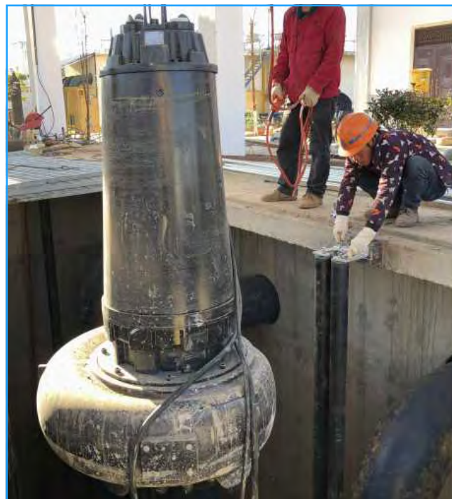
The UNIQA pump with cooling jacket lowered into the sump
