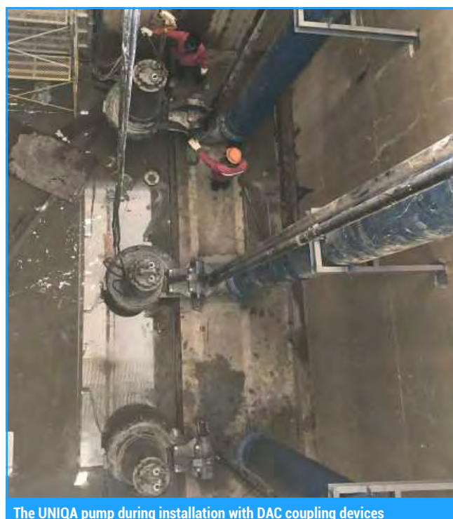
The UNIQA pump with cooling jacket lowered into the sump
