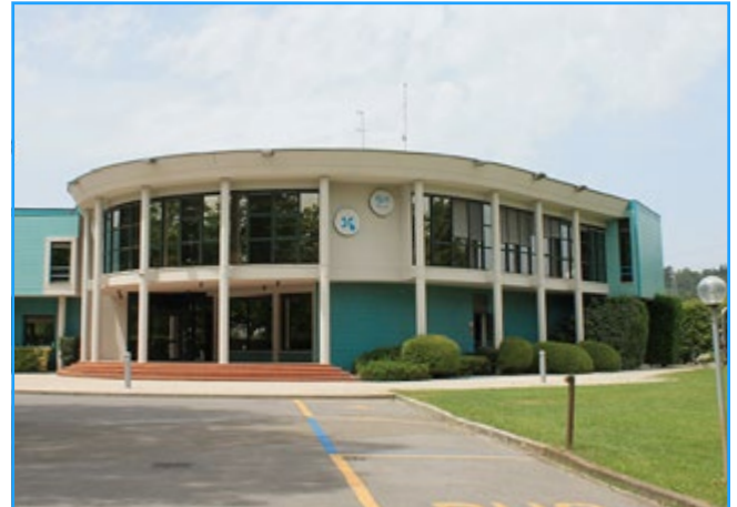
The headquarters of Consorzio Aquarno S.p.A.
