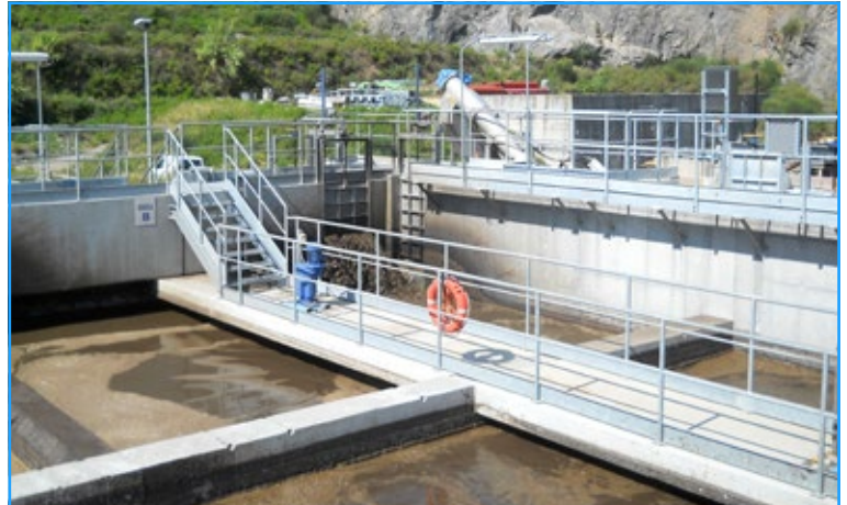
The waste water treatment facility
