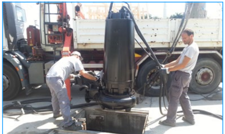
Pre installation phases
