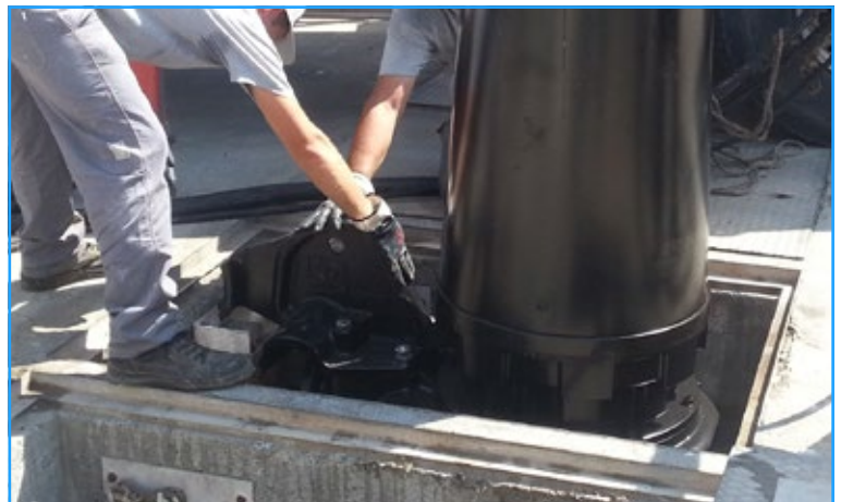
The installation of Zenit UNIQA in the sump
