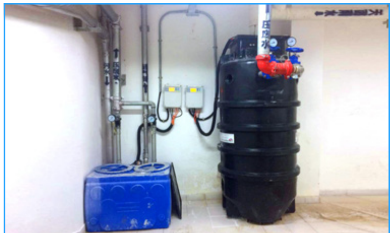
Pumping station installation
