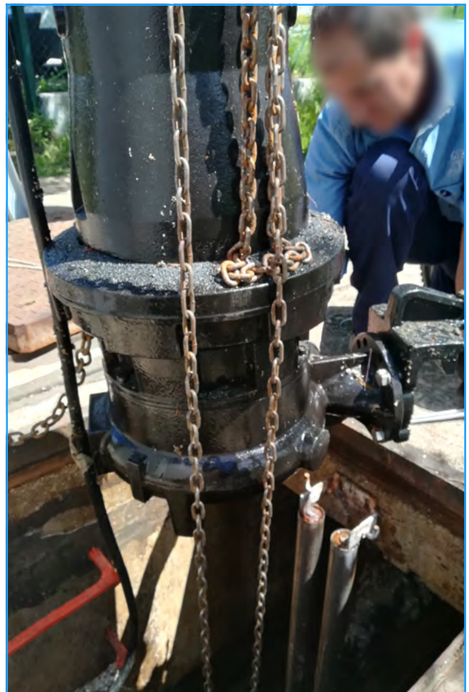
Installation of the UNIQA pump in the sump
