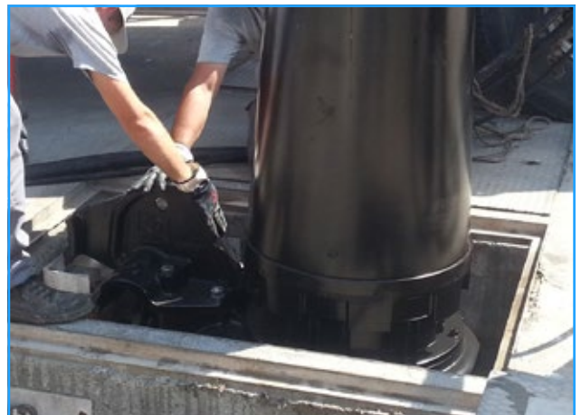
The installation of Zenit UNIQA in the sump
