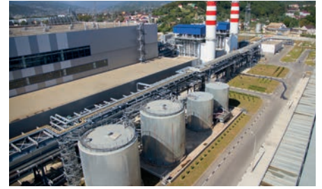
Electrical power plant
