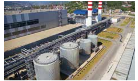
Electrical power plant
