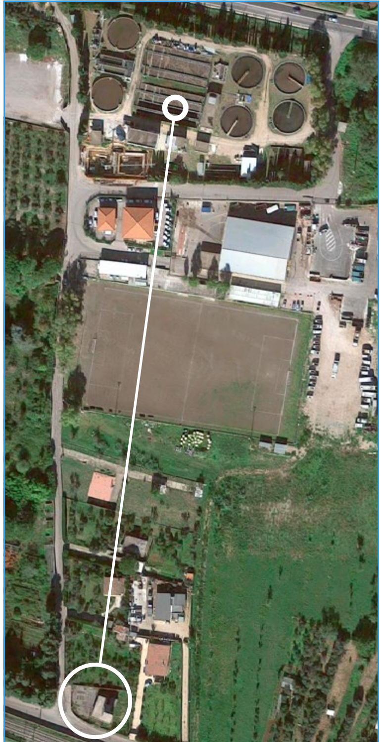
The lifting station and the wastewater plant
