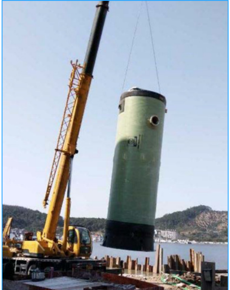
Tank hoisting
