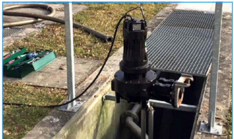
Pump ready to be lowered into the pit
