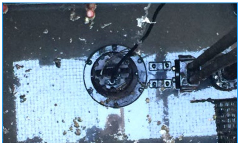
Pump ready to work
