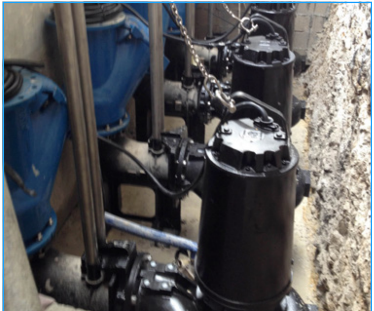
Pump installation into pumping station
