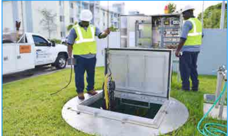
Mops sewage pump station with zenit uniqa pumps
